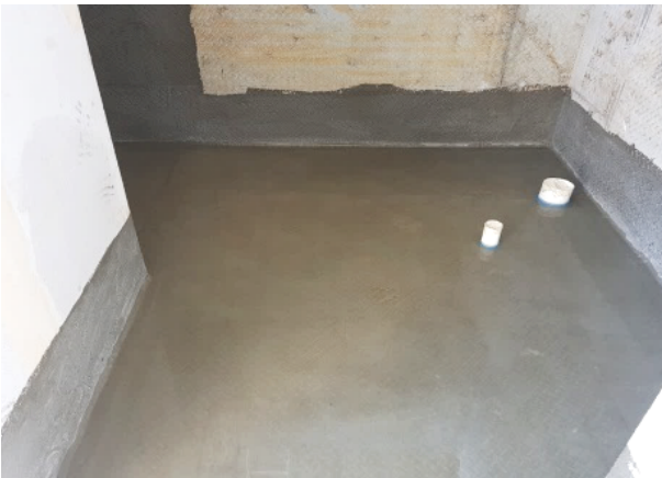
Figure: Water Ponding Test
