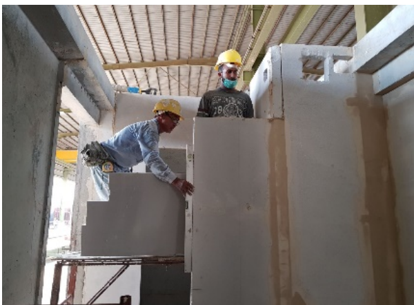
Figure: Lightweight Panel Installation
