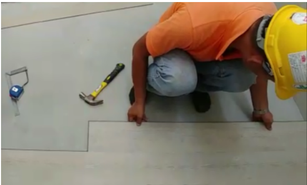
Figure: Floor finishes Installation
