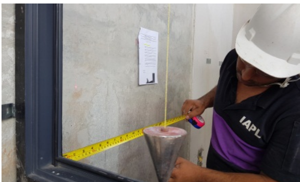
Figure: QC check on Window Installation
