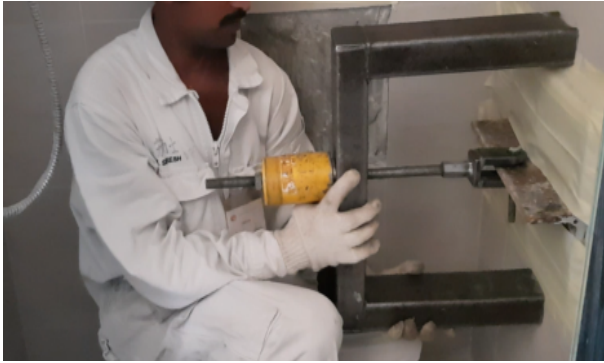
Figure: Alignment verification.
