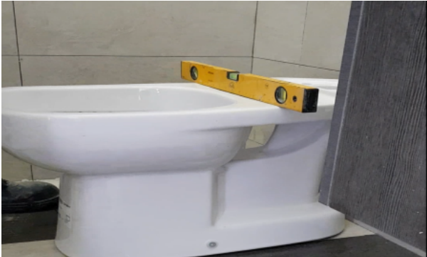
Figure: WC Installation
